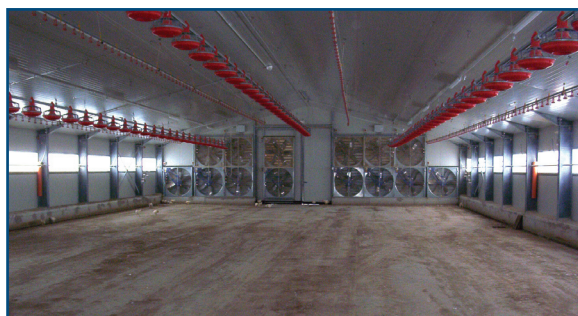
Figure 1. Chicken farming in an industrial broiler house: crosswise natural ventilation with windows and flap opening, specific longitudinal aeration system.
