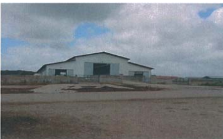
Figure 3 Control station (Bonassai)
