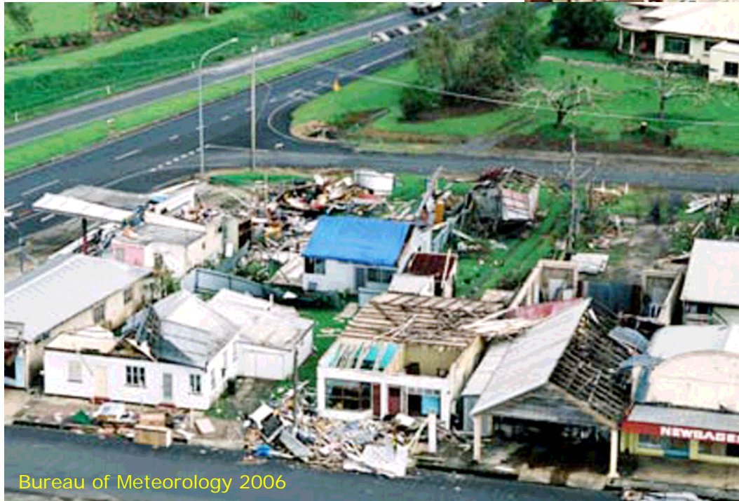
Damage to homes in Mourilyan
