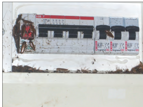
Figure 4 Infested electrical control panel after application of insecticide gel
