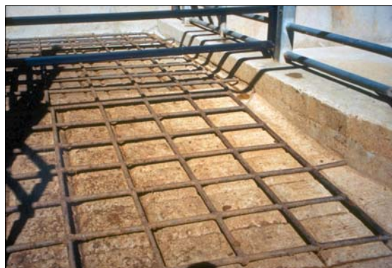
Figure 4 A mat of welded steel rods can be used to provide a non-slip surface on scales and other high traffic areas with worn out slick floors. The bars must never be criss-crossed; they must be cut so they will lie flat on the floor.
