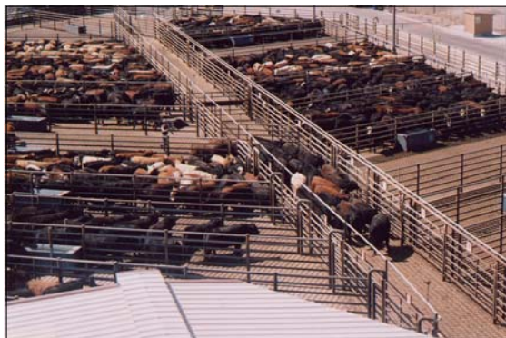
Figure 6 A holding yard with two rows of diagonal pens laid out on a 60° angle Animals unloaded from trucks move into the pens through the outer alleys and leave the pens through a central alley A 70°-80° angle can also be used; do not use a steep 45° angle
